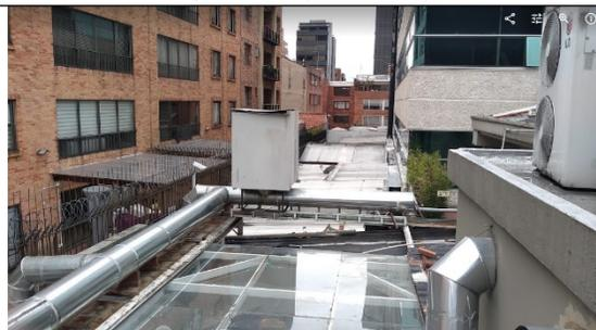
FOTO No. 4 EXTRACTOR Y SISTEMA DE DUCTOS
